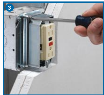
Re-tighten... Adjustment screws.
